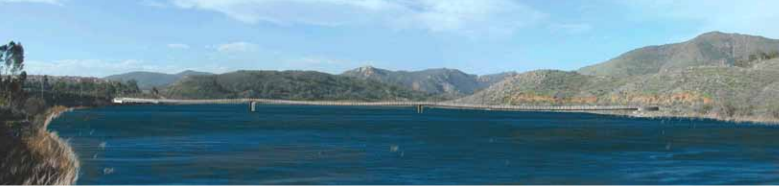
An early rendering of the David Kreitzer Lake Hodges Bicycle Pedestrian Bridge illustrates its appearance "floating" above the water.
