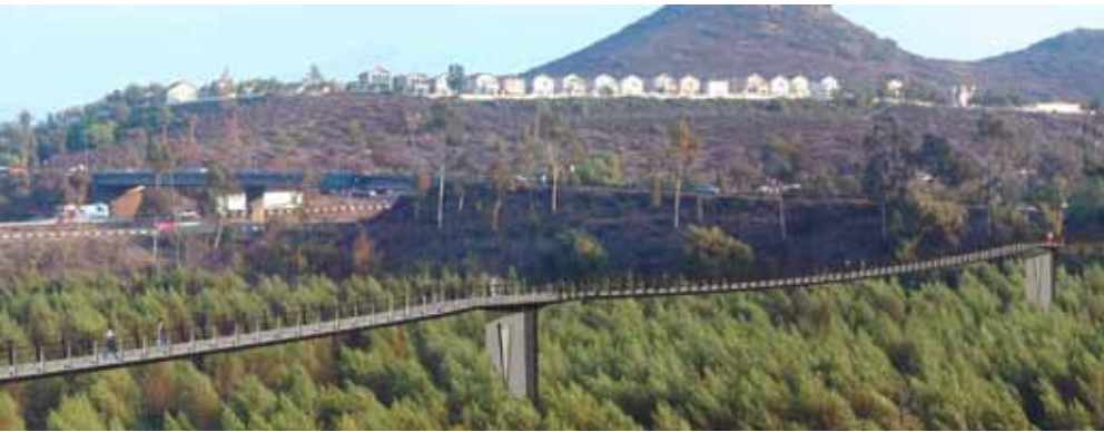
In the dry condition, the bridge appears to "nest" above the trees.
