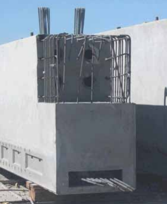
Girder end zones required strut-and-tie techniques during design to provide more reliable, economical details.
