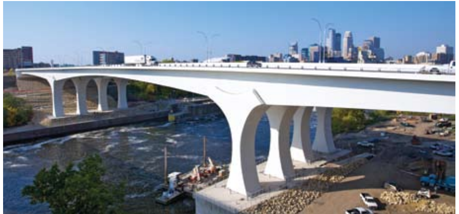
The I-35W St. Anthony Falls Bridge used combinations of fly ash, slag, and silica fume in the different concrete mixes. Photo courtesy of FIGG, Tim Davis photographer.
