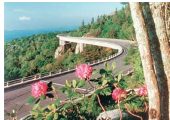
Blue Ridge Parkway Viaduct was built from the top down and incorporated iron oxide pigments in the concrete to minimize environmental impact. Photo courtesy of FIGG.
