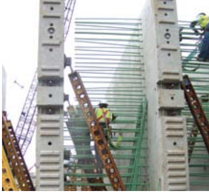
The diaphragms between beam lines used epoxy-coated reinforcement. Photo: Cianbro Corp.
