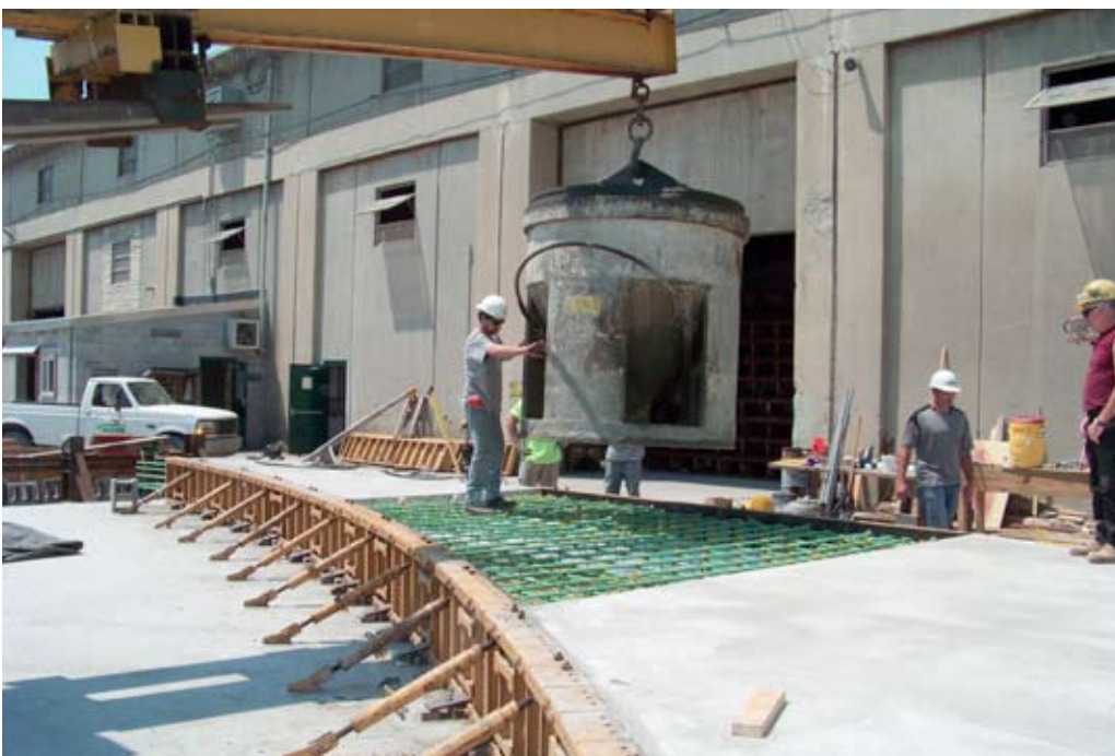
The precast concrete arches had a complicated series of temporary post-tensioning and sequenced permanent post-tensioning procedures to follow. The strand and reinforcing bar layouts within the components were complex. Photo: Northeast Prestressed Products LLC.
