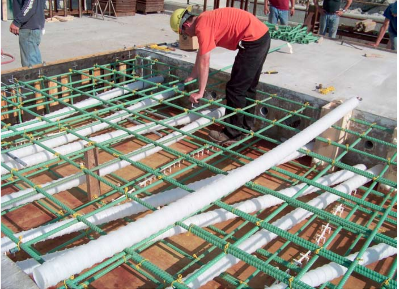
The precast concrete arches had a complicated series of temporary post-tensioning and sequenced permanent post-tensioning procedures to follow. The strand and reinforcing bar layouts within the components were complex. Photo: Northeast Prestressed Products LLC.
