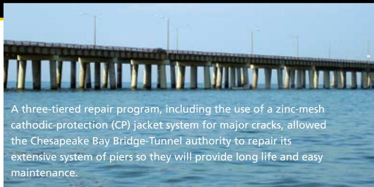
A three-tiered repair program, including the use of a zinc-mesh cathodic-protection (CP) jacket system for major cracks, allowed the Chesapeake Bay Bridge-Tunnel authority to repair its extensive system of piers so they will provide long life and easy maintenance.
