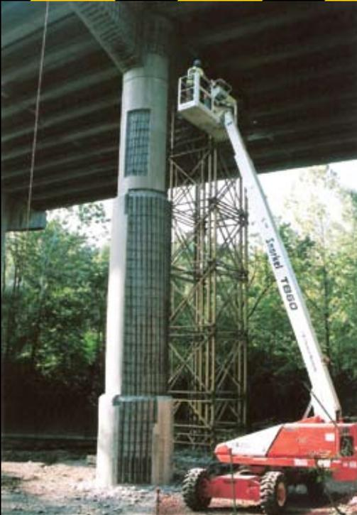
A drymix shotcrete process was used to repair the badly deteriorated piers on the Noblestown Road Bridge near Pittsburgh, Pa. The repair method allowed the bridge to remain open during construction and return to full operation quickly.
