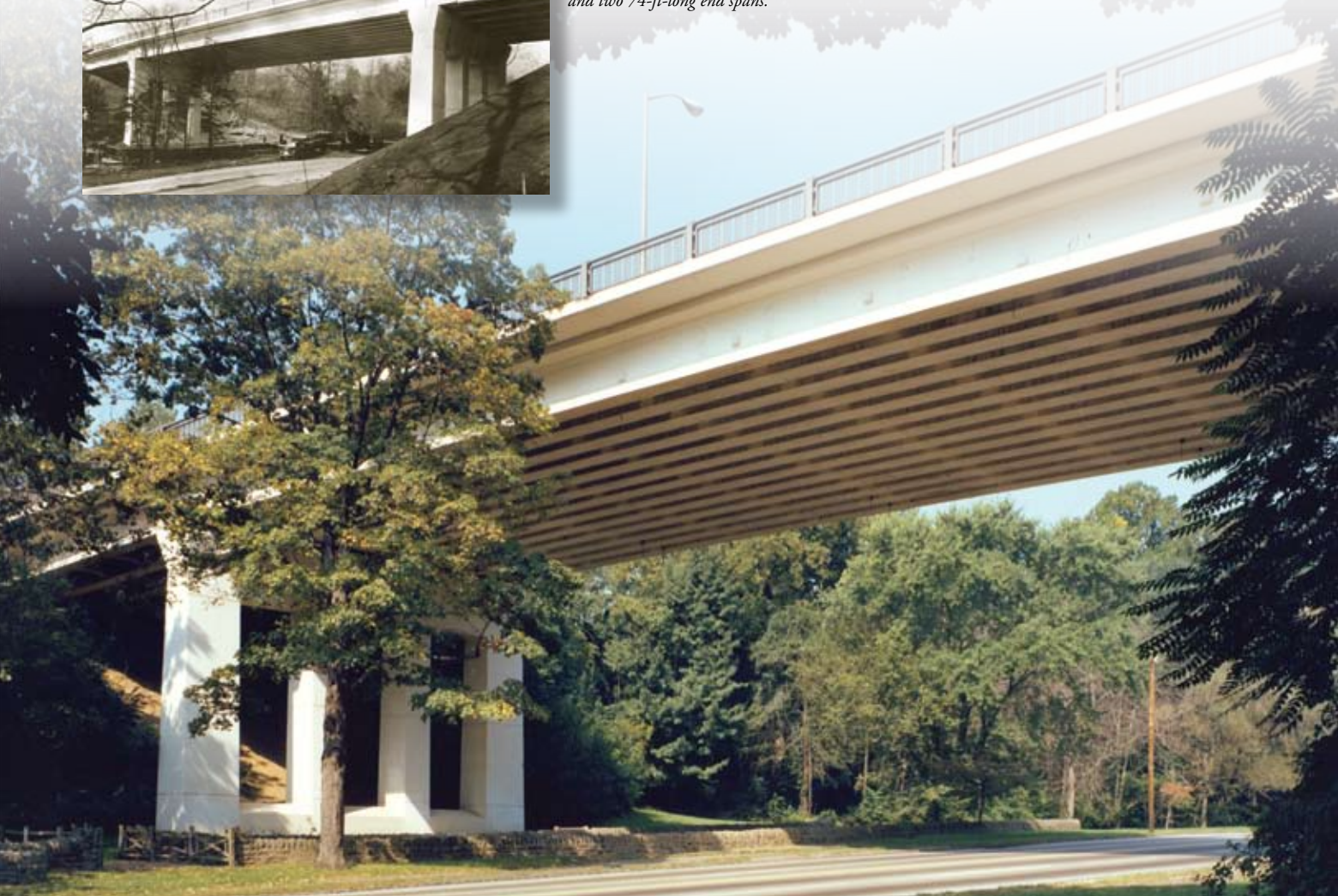
The first major prestressed concrete bridge in America was constructed in Pennsylvania in 1950. Using concepts devised by Professor Gustave Magnel of the University of Ghent in Belgium, the Walnut Lane Bridge in Philadelphia features a 160-ft-long main span and two 74-ft-long end spans.
