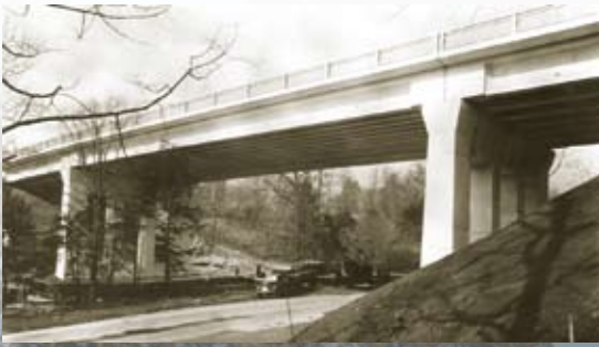
The first major prestressed concrete bridge in America was constructed in Pennsylvania in 1950. Using concepts devised by Professor Gustave Magnel of the University of Ghent in Belgium, the Walnut Lane Bridge in Philadelphia features a 160-ft-long main span and two 74-ft-long end spans.
