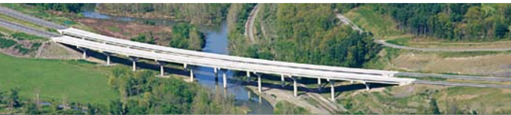
The Tioga River Bridge on Route 15 features twin, 11-span structures constructed with precast, prestressed concrete I-beams. The $26.9-million project connects two key roadways to speed traffic flow and accessibility in Lawrenceville, Pa.
