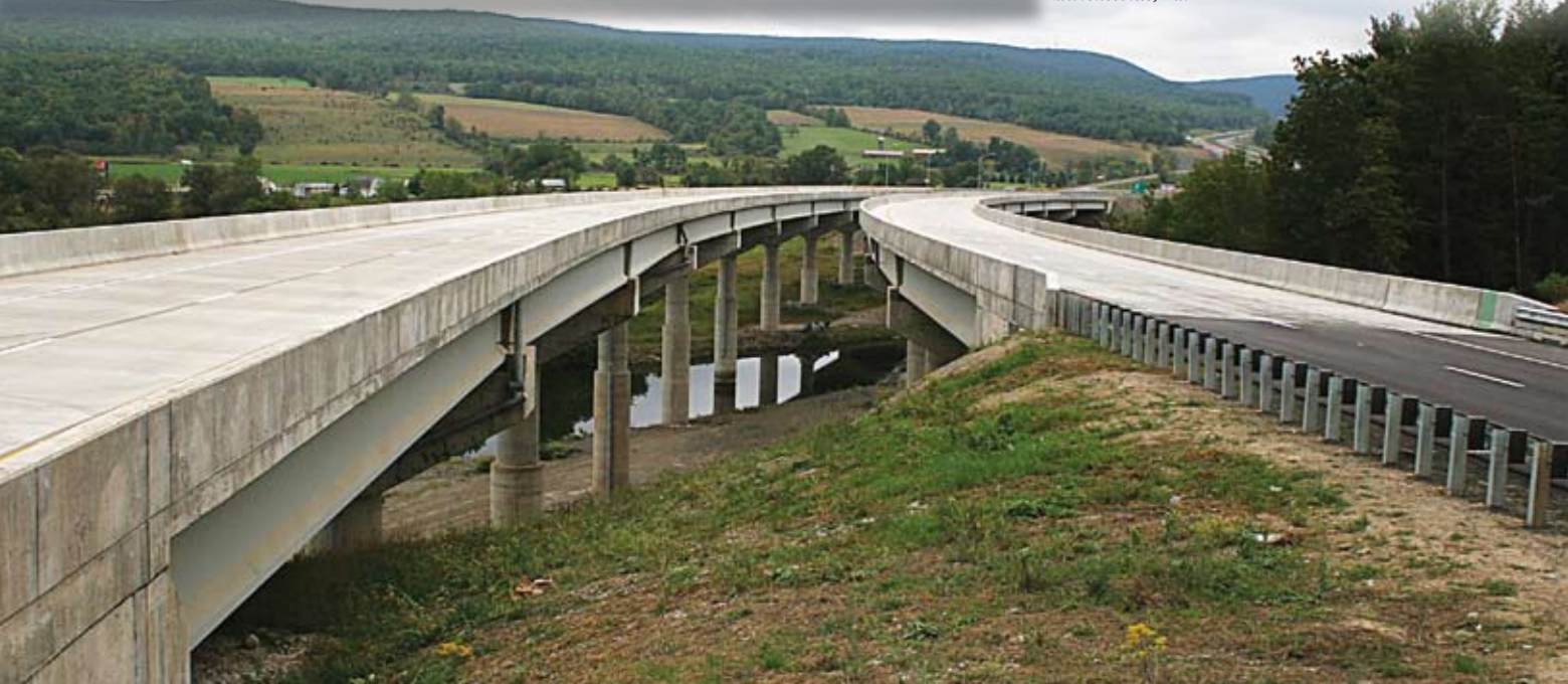
The Tioga River Bridge on Route 15 features twin, 11-span structures constructed with precast, prestressed concrete I-beams. The $26.9-million project connects two key roadways to speed traffic flow and accessibility in Lawrenceville, Pa.
