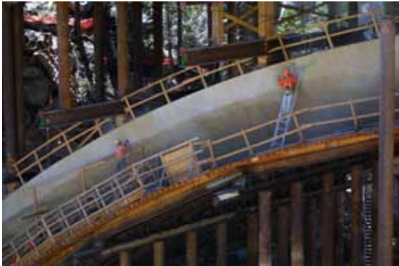
Finishing work proceeds on one of the concrete arches.
