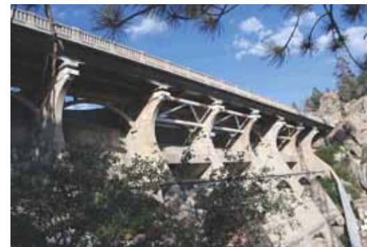
The Big Bear Dam and existing bridge.
