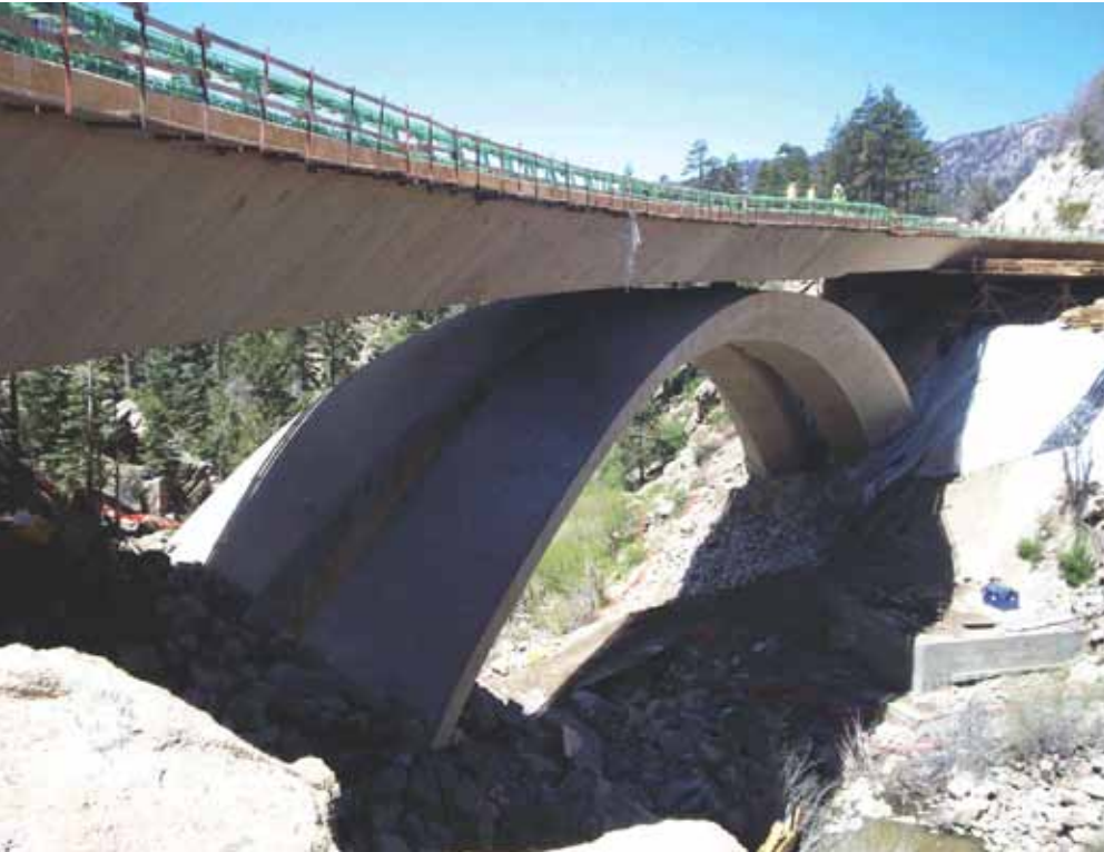
The Big Bear Bridge nears completion.
