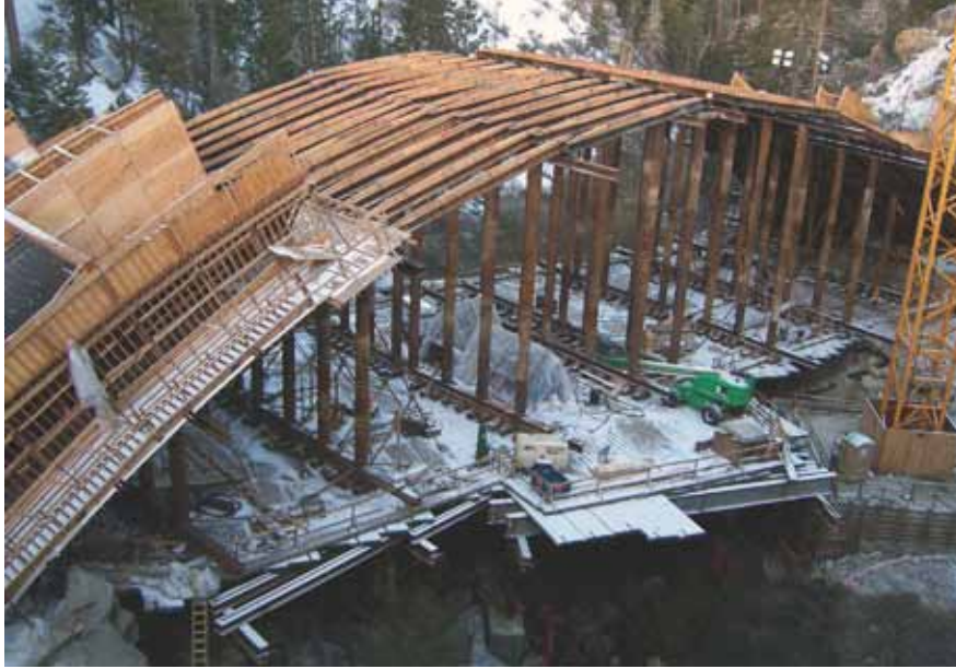
Falsework and forming for the arches.
