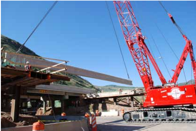
Placing AASHTO Type II beams on the temporary abutments.
