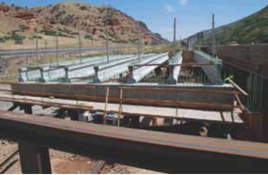
Beam erection is complete on the temporary abutment.
