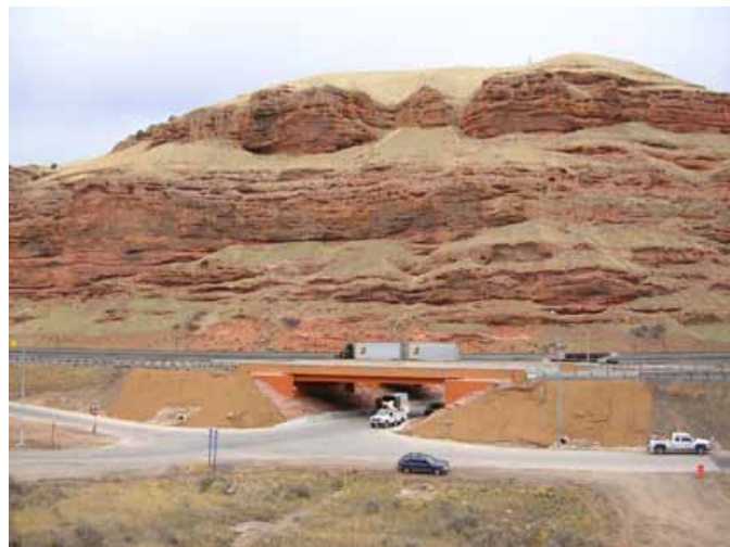
The aesthetic scheme for the new bridges was in keeping with the surrounding red rock cliffs and desert landscape.
