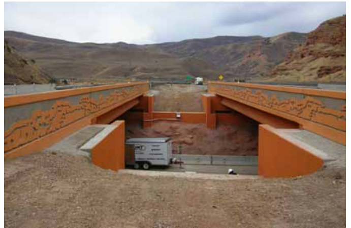
View of the completed I-80 Bridges over Echo Dam Road.
