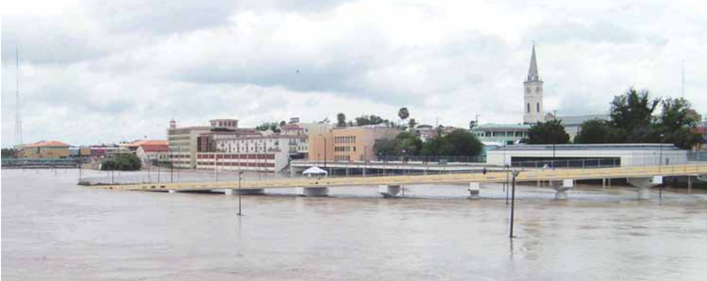
Less than a year after completion, the Rio Grande River submerged the bridge under 23 ft of water during a flood in July 2010.
