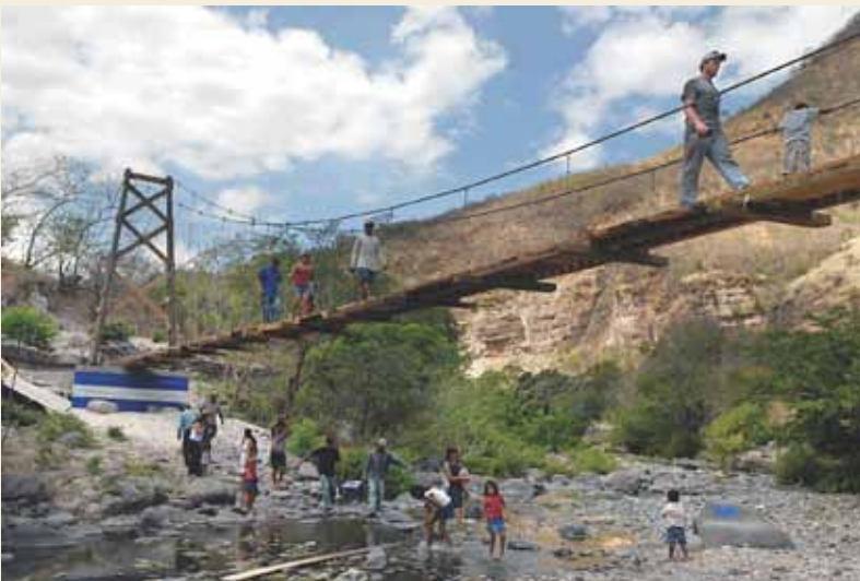
McNary Bergeron's work with Bridges to Prosperity Inc. has included La Pintada suspension footbridge in Honduras. This bridge connects four formerly inaccessible communities. The firm helped design the structural towers that support the bridge on the low-lying plain, which had been an obstacle to creating the bridge previously.
