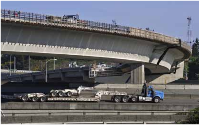
The Nalley Valley Interchange on I-5 through Tacoma, Wash., represents one of the few value-engineering projects that McNary Bergeron has done. The two bridges were redesigned from steel tub-girders to a precast concrete segmental box-girder design. The change reduced costs while maintaining the original alignment.
