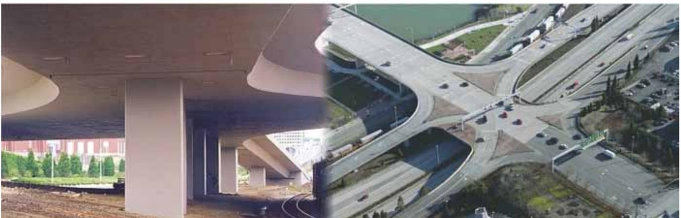
On the State Route 509 interchange that spans I-705 and the BNSF Railway track in Tacoma, Wash., BergerABAM created a curving, elevated single point urban interchange, the first in Washington state and one of the first in the country. The structure features cast-in-place, post-tensioned concrete box girders with variable-depth webs.
