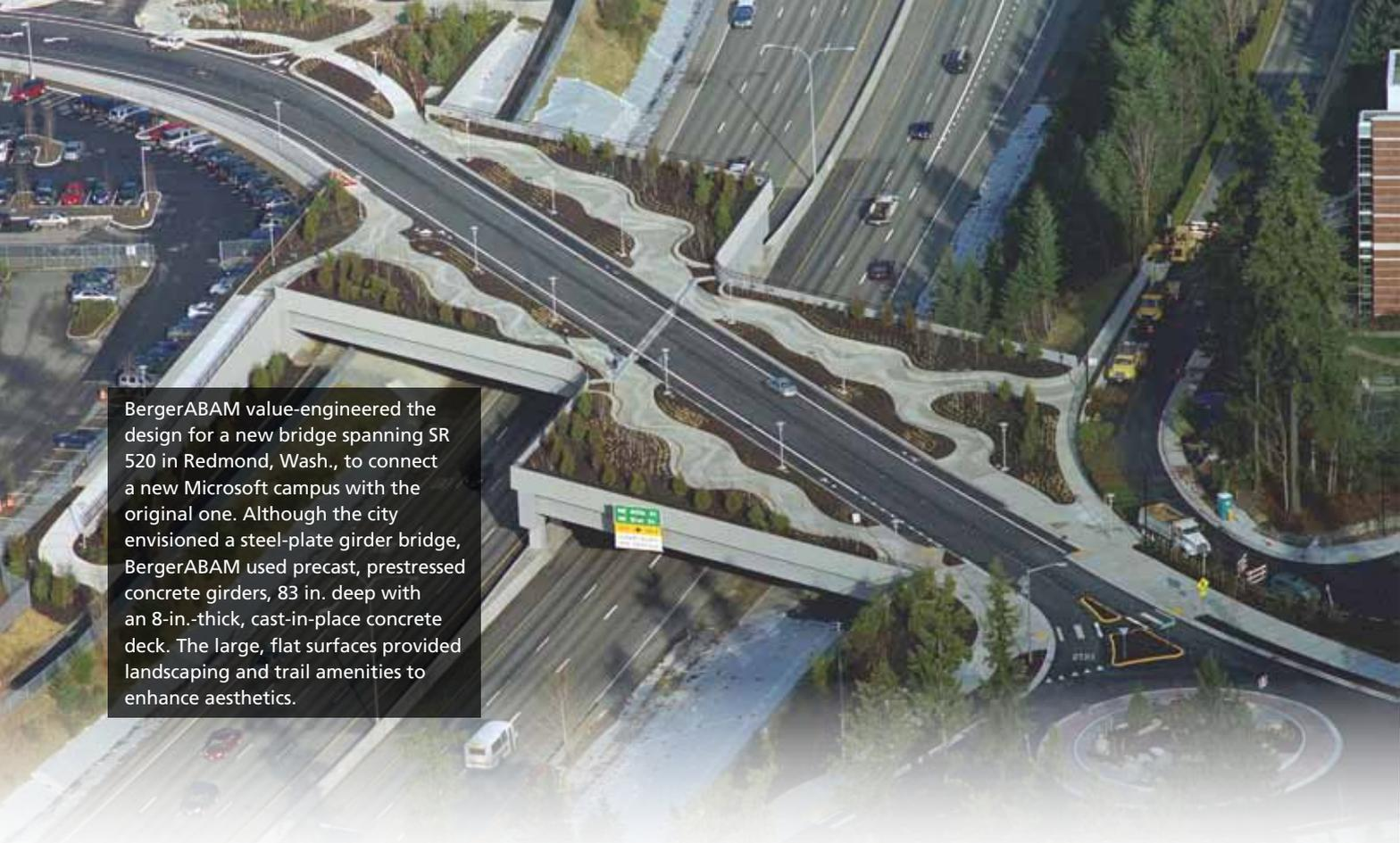
BergerABAM value-engineered the design for a new bridge spanning SR 520 in Redmond, Wash., to connect a new Microsoft campus with the original one. Although the city envisioned a steel-plate girder bridge, BergerABAM used precast, prestressed concrete girders, 83 in. deep with an 8-in.-thick, cast-in-place concrete deck. The large, flat surfaces provided landscaping and trail amenities to enhance aesthetics.
