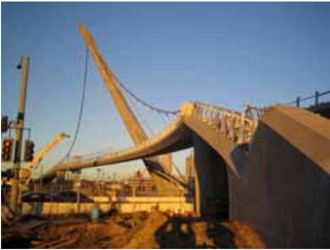
The main cables extend to the base of the stairs and anchor in the abutments. The angle change from the deck to the stairs is accommodated by a steel deviator placed at the top of each stair span and embedded in the concrete bent cap.
