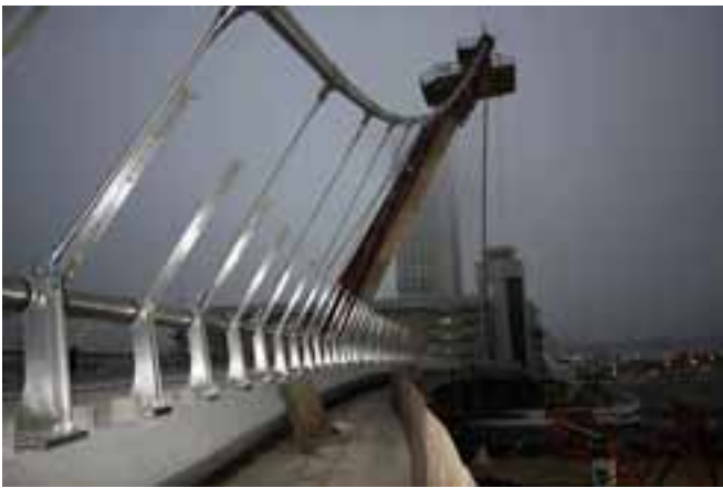
The main cables extend to the base of the stairs and anchor in the abutments. The angle change from the deck to the stairs is accommodated by a steel deviator placed at the top of each stair span and embedded in the concrete bent cap.
