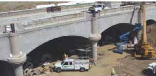
Placement of balustrade railings on beam face projections and architectural precast concrete pilasters on the edges of bents 2, 3, and 4. Photo: City of Rancho Cucamonga.
