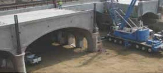
Fascia beams with vertical face projections are 2.45 ft deeper providing confinement for the roadbed ballast and a base for the balustrade railings. Photo: PBS&J, an Atkins company.
