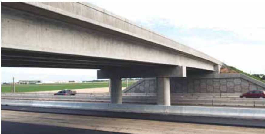
Precast concrete bent caps and columns were used on the Robinson Road over I-84 Bridge, one of several recent projects to incorporate accelerated bridge construction (ABC) techniques.
