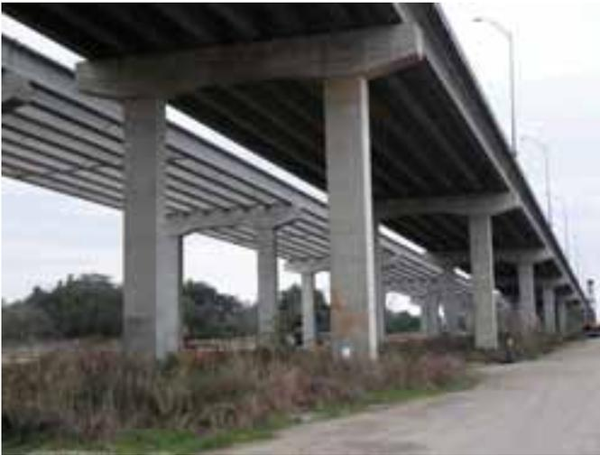
Approach spans for the Trinity River Bridge ranged from 116 ft to 150 ft and used precast, prestressed concrete AASHTO Type VI beams.
