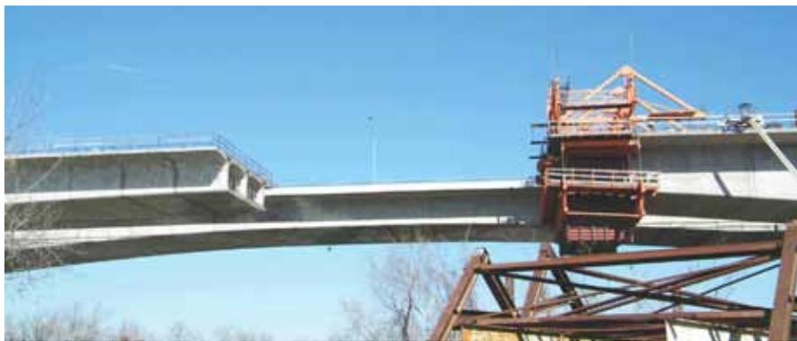
Nearing closure of the 450-ft-long main span of the eastbound bridge. The girder is 10.5 ft deep at midspan.
