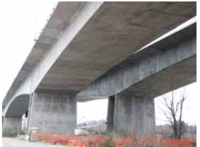
The Trinity River Bridge has cast-in-place concrete flared, double wall piers.
