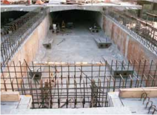
One cell of the twin cell box girder showing the post-tensioning anchorage blisters for the continuity tendons. Forming is being installed for the deck closure pour between the ends of the main span cantilevers.
