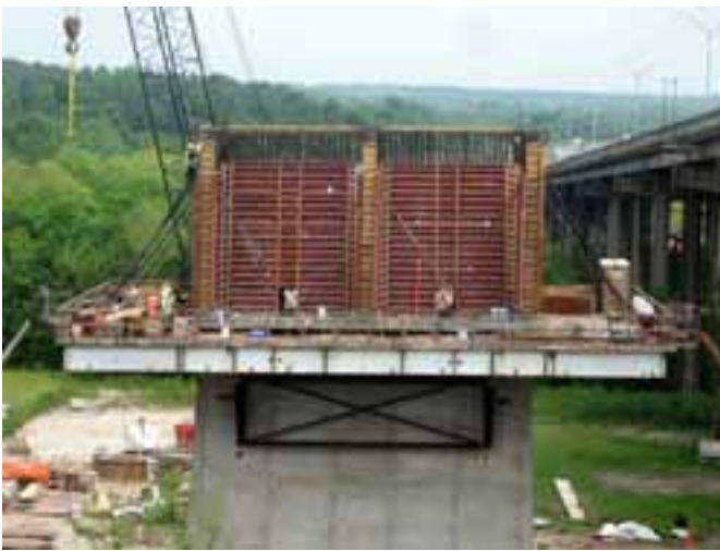
Forming of the inclined pier segment diaphragms in the twin cell box girder that is 25 ft deep at the pier and the pier segment after casting.
