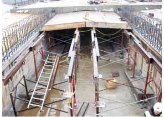
One cell of the twin cell box girder showing the post-tensioning anchorage blisters for the continuity tendons. Forming is being installed for the deck closure pour between the ends of the main span cantilevers.
