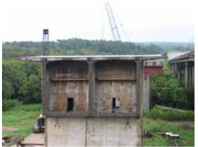
Forming of the inclined pier segment diaphragms in the twin cell box girder that is 25 ft deep at the pier and the pier segment after casting.
