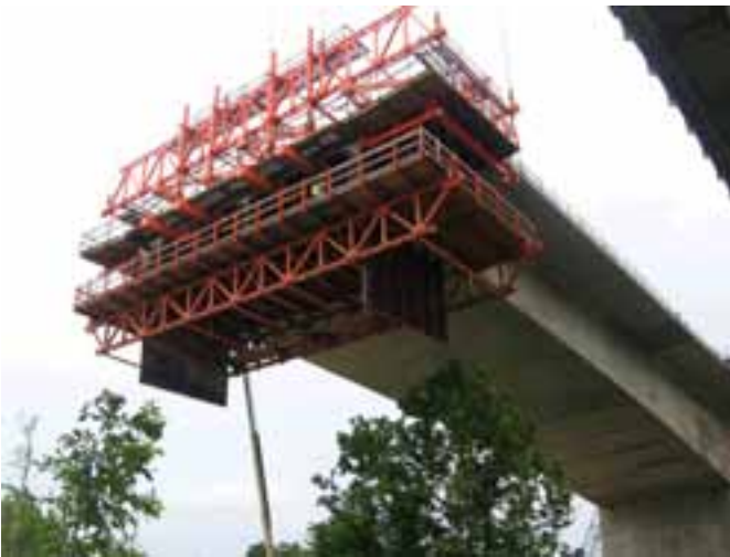
A form traveler was used to cast the 15-ft 6-in.-long segments.
