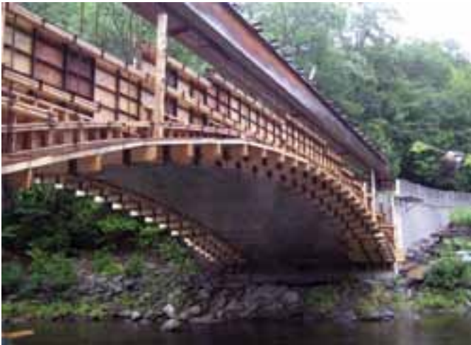
The arch forming system was designed to keep falsework out of the river. The tie rods supporting the forms were adjusted during the casting to keep the form stationary while the beam deflected. Photo: C. D. Davenport.
