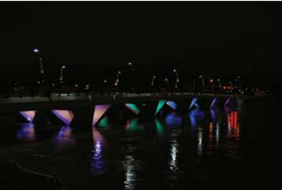
Custom-designed lanterns are nested in extensions of the sloping pier walls on the Cypress Avenue Bridge.
