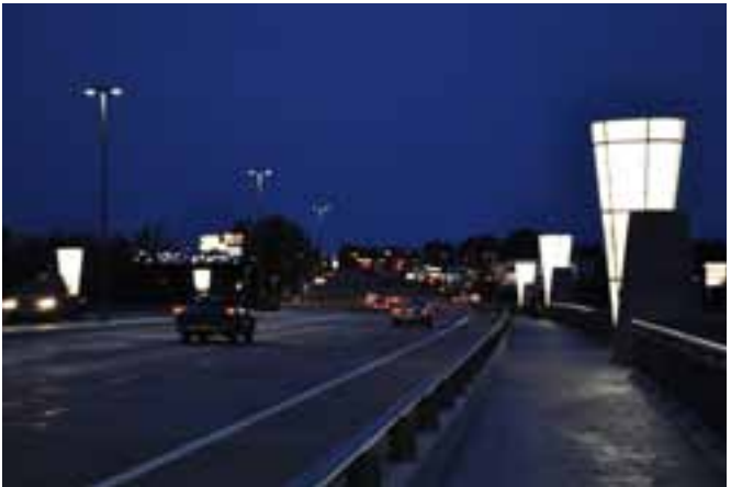
Custom-designed lanterns are nested in extensions of the sloping pier walls on the Cypress Avenue Bridge.
