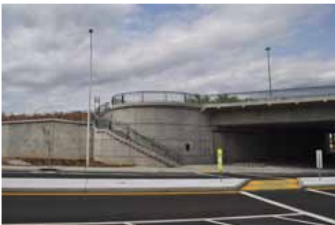
Abutment overlook with spiral-shaped stairway extends to Park Marina Drive, a frontage road along the Sacramento River. Photo: C. Hodge, T.Y. Lin International.
