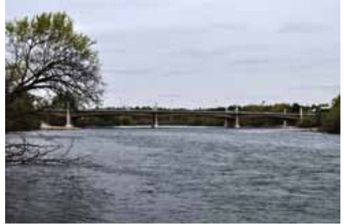
The shallow, gently-arched soffit connects the riverbanks during the day. Photo: C. Hodge, T.Y. Lin International.
