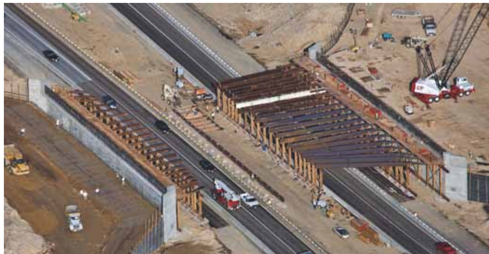
Falsework construction had minimal impacts to I-84 motorists. Photo: Idaho Airships.
