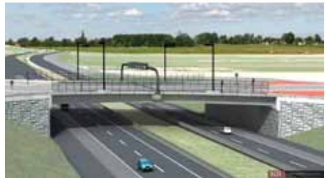
Custom formliners used along parapets and walls. Photo: HDR Inc.
