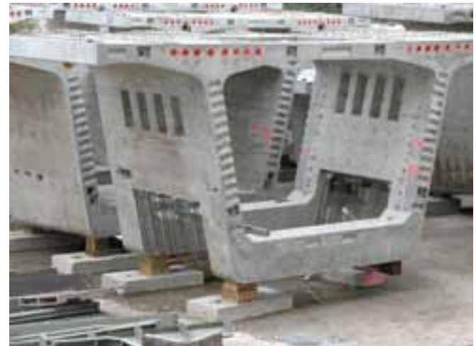
A dual-track precast concrete pier shell segment. Photo: URS Corporation.
