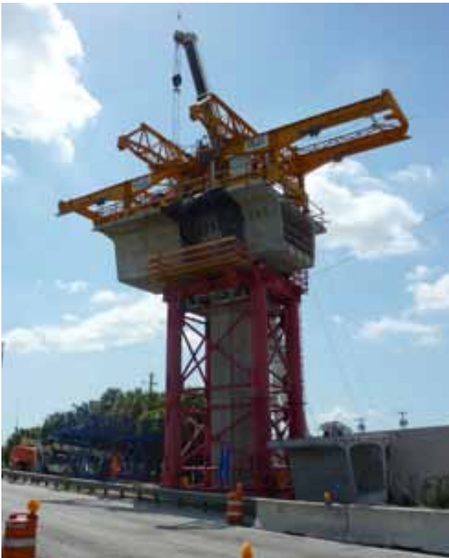
A dual-track expansion pier diaphragm segment showing the expansion joint face. Photo: Rizzani de Eccher USA.
