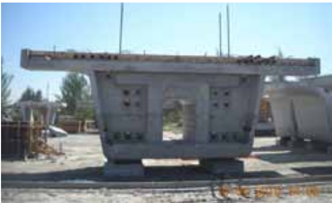
A dual-track expansion pier diaphragm segment showing the expansion joint face. Photo: Rizzani de Eccher USA.
