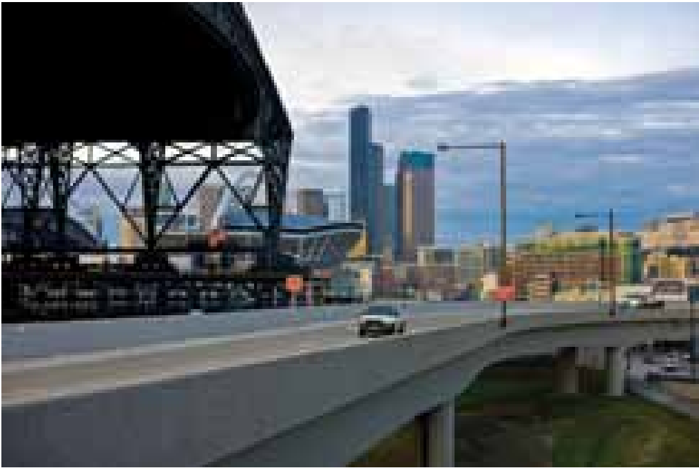
With downtown Seattle as the backdrop, traffic sweeps along the new Atlantic Ramp Bridge, a traditional cast-in-place, post-tensioned concrete box girder bridge. Photo: John Livzey.
