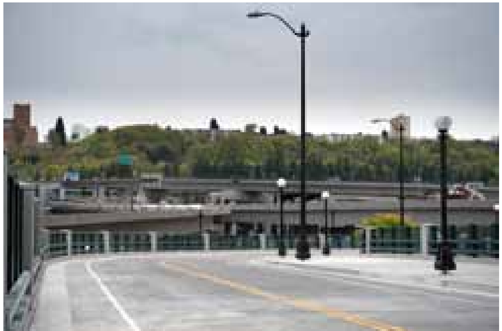
With its 5-ft bike lanes and 18-ft-wide sidewalk, the new Royal Brougham Bridge now separates bicyclists and pedestrians from the hazards posed by train traffic. Photo: Washington State Department of Transportation.
