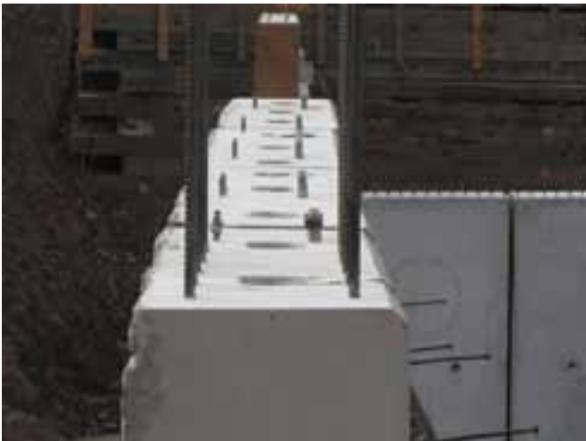
The top edges of the wingwalls had provisions to mount the rail posts and attach the cast-in-place concrete end block. Photo: Hoyle, Tanner & Associates Inc.
