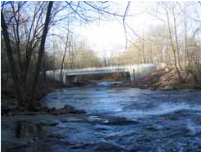
The final adjacent box beam was set on the precast concrete beam seat after which the cheek walls were set. Epoxy-coated reinforcement was provided in the tops of the box beams to secure the curbs and sidewalks. Photo: Arborio Corporation.
