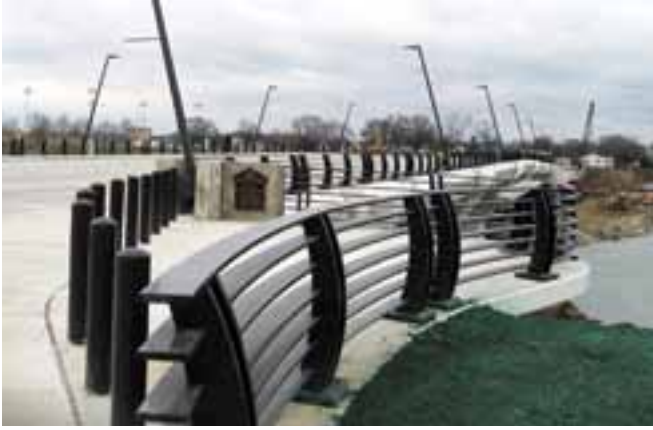
Curvilinear rail and cantilever slab frame an overlook and view of the Great Miami River. Photo: Woolpert Inc.
