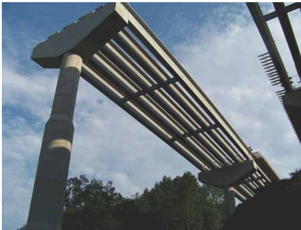
Careful selection of span lengths was needed to place piers to avoid impacting the river, creek, historic canal, railroad tracks, and access road.
