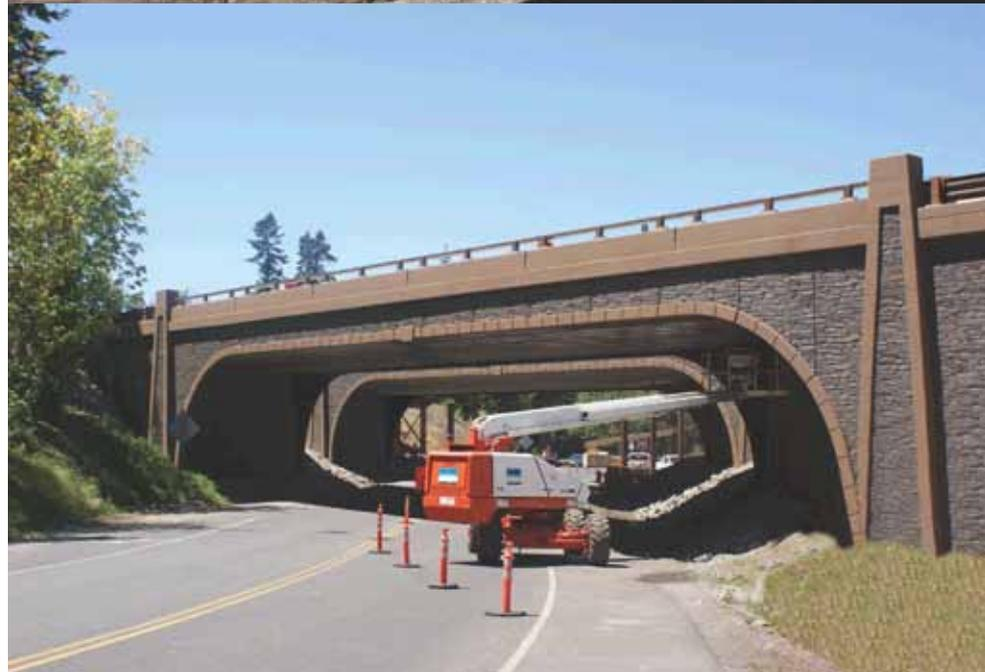
*The guidelines in Oregon's I-84 Corridor Strategy emphasize a Cascadian bridge style that features precast concrete panels with a façade cast on textured formliners. Designers must pay close attention to the connections for such panels to ensure they fit in the field. Photos: Knife River Corp.*
