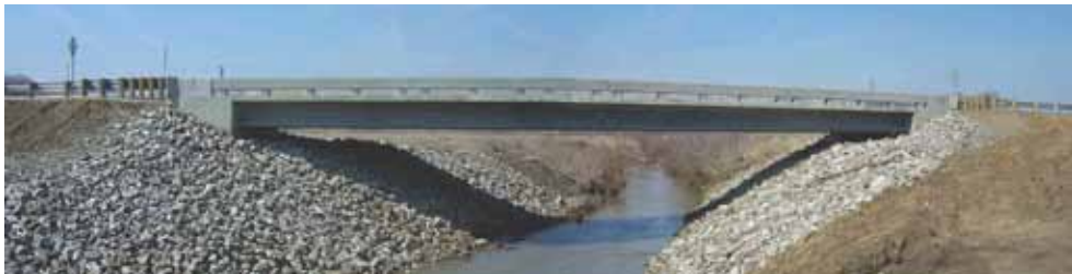
Wapello County's first bridge to be built with UHPC was the Mars Hill Bridge. It features three 110-ft-long precast, prestressed concrete, 45-in.-deep Iowa bulb-tee beams topped with a cast-in-place concrete deck.
