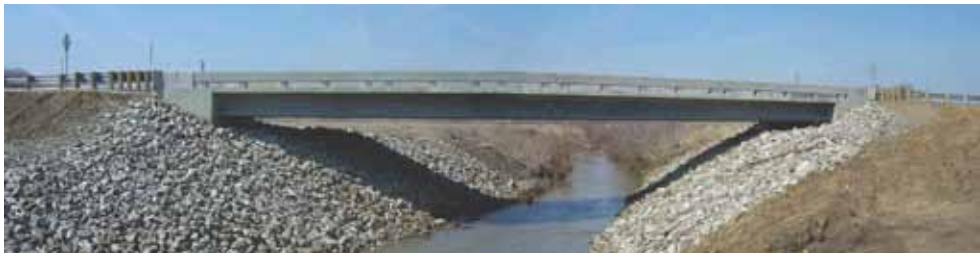
Wapello County's first bridge to be built with UHPC was the Mars Hill Bridge. It features three 110-ft-long precast, prestressed concrete, 45-in.-deep Iowa bulb-tee beams topped with a cast-in-place concrete deck.
