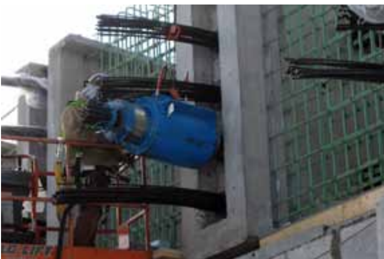
After splices were cast and cured, each of five tendons was pulled to approximately 960 kips. Photo: VHB—Vanasse Hangen Brustlin Inc.
