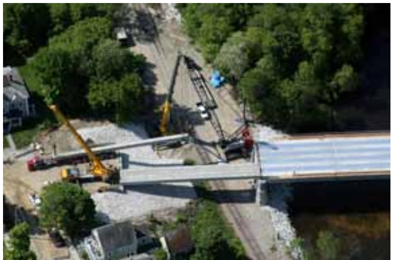
Span 3 box beams were erected through a sequence of carefully choreographed crane movements. In this photo, one crane passes the end of a box beam to another crane for final placement. Photo: VHB—Vanasse Hangen Brustlin Inc.
