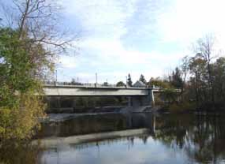
The Cross Street Bridge nearing completion. Photo: VHB—Vanasse Hangen Brustlin Inc.
