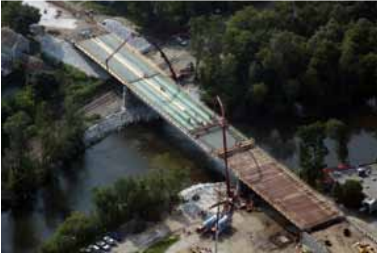
A crew places the cast-in-place concrete deck. Photo: VHB—Vanasse Hangen Brustlin Inc.
