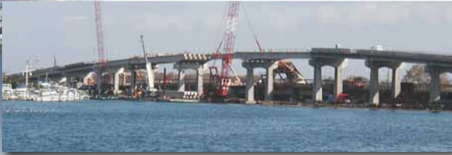
The new $43 million precast concrete bridge along Route 35 over the Shark River in Belmar, N.J., extends 2000 ft using 17 spans of AASHTO girders, including a main span of 170 ft. The bridge, which replaced a bascule bridge that disrupted traffic to beachfront communities, is 84 ft wide and carries four lanes of traffic.
