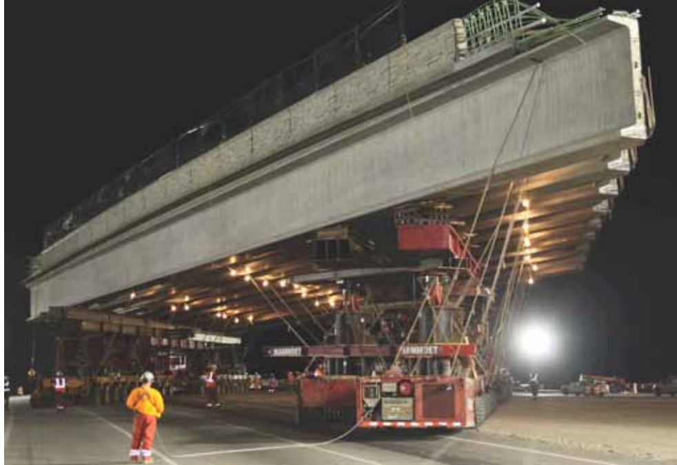
Bridge span on the move during 8-hour road closure.
