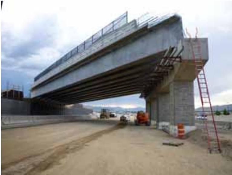
First span of the eastbound bridge placed in its final location.
