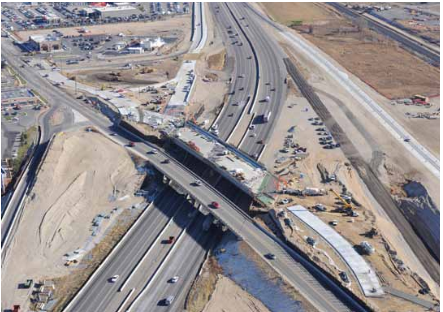
Work being completed on the Phase 1, westbound bridge. Traffic was maintained on the existing structure prior to being moved to the spans placed during Phase 1.
