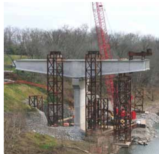
Temporary towers supported steel beams spanning over the piers that in turn supported a gantry with strand jacks to lift the pier segments and move them laterally into place. Photo: Haydon Bridge Co.
