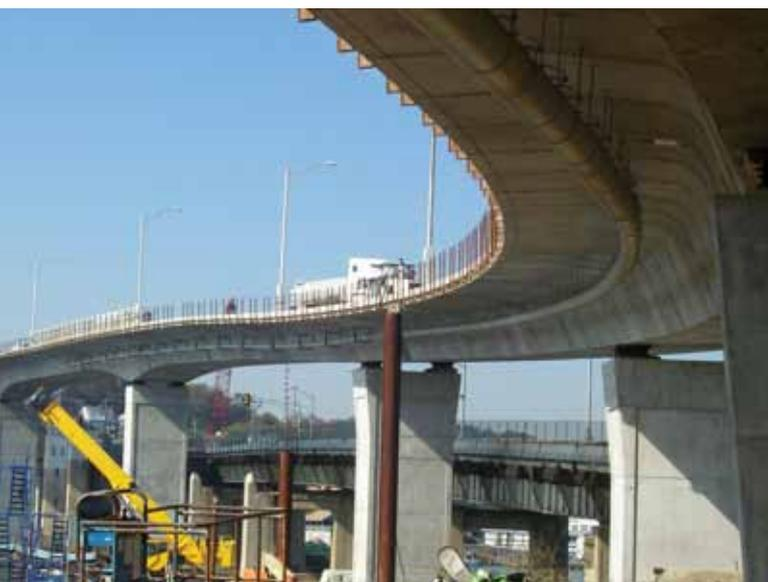
Precast concrete footings, piers, and superstructure segments were used to accelerate construction on the Route 36 Highlands Bridge. Photo: J. H. Reid General Contractor, Unistress Corporation, or DYWIDAG-Systems International USA Inc.
