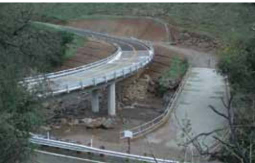
Looking north at the completed Black Canyon Road Bridge and the original structure. The original structure will be used by non-motorized traffic. Photo: County of San Diego.
