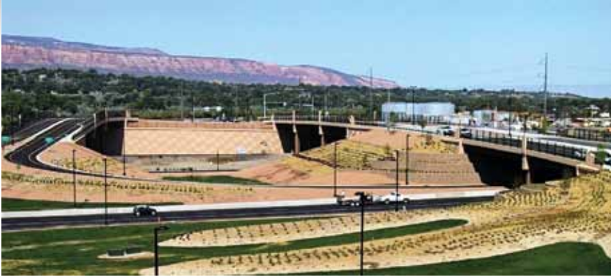
The $110-million Riverside Parkway project (shown here during the 2008 Grand Opening) required three bridges at the U.S. Highway 50 crossing. Two carry the parkway over the Union Pacific Railroad tracks and the third bridge connects the on/off ramps to U.S. Highway 50. All photos: Grand Junction, Colo.
