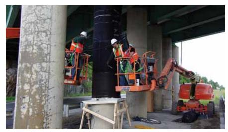
Application of Carbon Fiber Reinforcement Polymer (CFRP) wrap to a bridge column. Photo: Federal Highway Administration.
