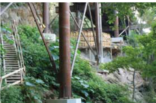
View below the temporary work trestle, as pier 1 footing is formed on top of the sub-footing concrete.
