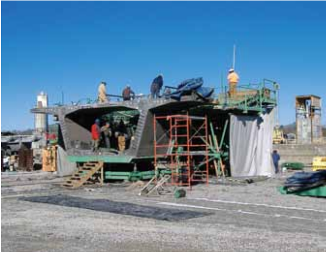
Precast segments were cast using the short-line casting method. All photos: Federal Highway Administration.
