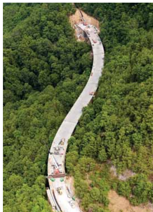
Completed construction of the major bridge elements.
