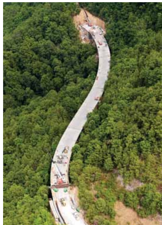
Completed construction of the major bridge elements.
