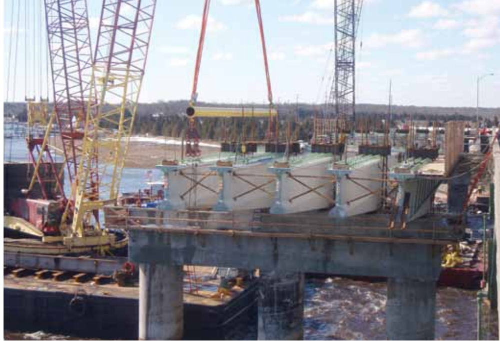
Pier 1 segment installation.
