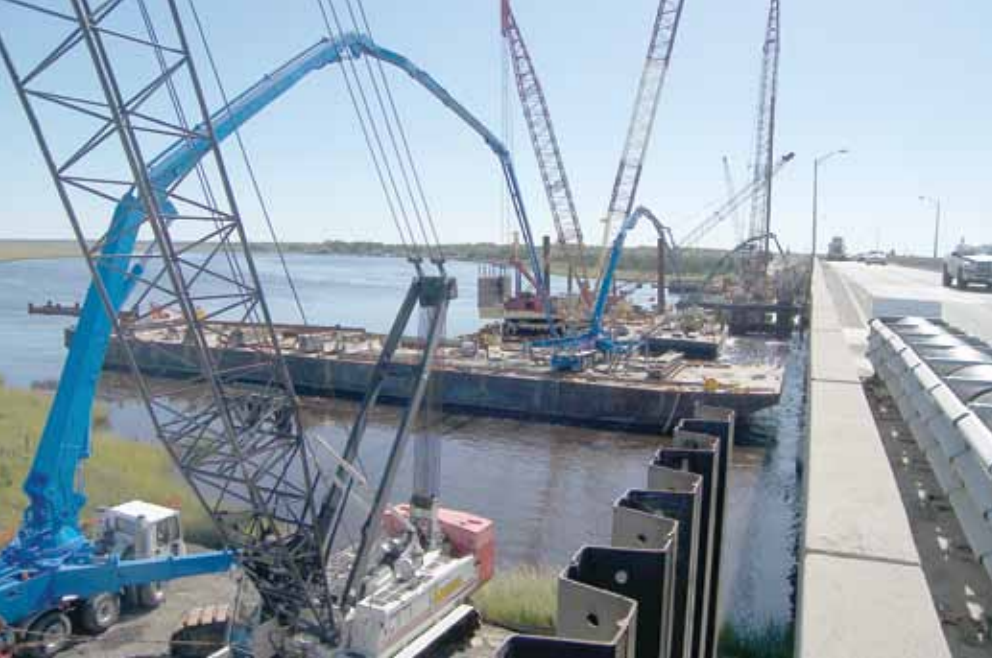
Concrete pumping trucks were used in series to install the self-consolidating concrete in the drilled shafts.
