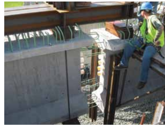
Span segment installation with strong-backs.
