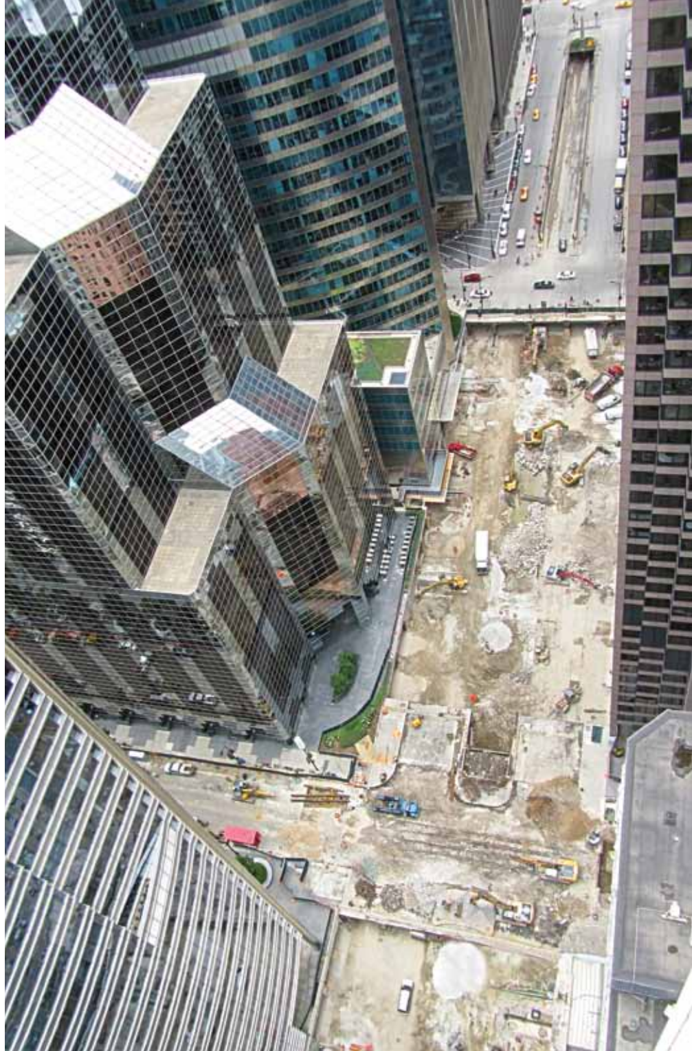
View from adjacent skyscraper looking down on the existing Madison Street intersection prior to completing deck demolition. Photo: McHugh Construction.
