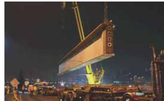
A 125-ft-long segment is being erected in Span 1.
