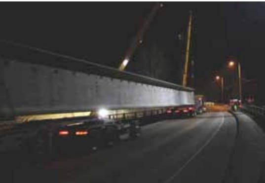
One of the longest girder segments at 125 ft is shown being transported to the site during nighttime erection to reduce impact to traffic.
