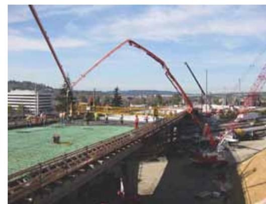
Epoxy-coated reinforcing steel was used to extend the life of the cast-in-place concrete deck.
