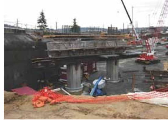
Pier 2 nears completion of its column beam. Seismic isolation casings can be seen around the columns just above the ground.
