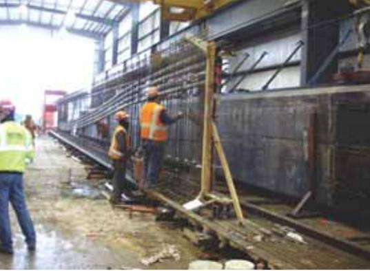
The 8-ft 4-in.-deep girder is shown during production in the precast production building.
