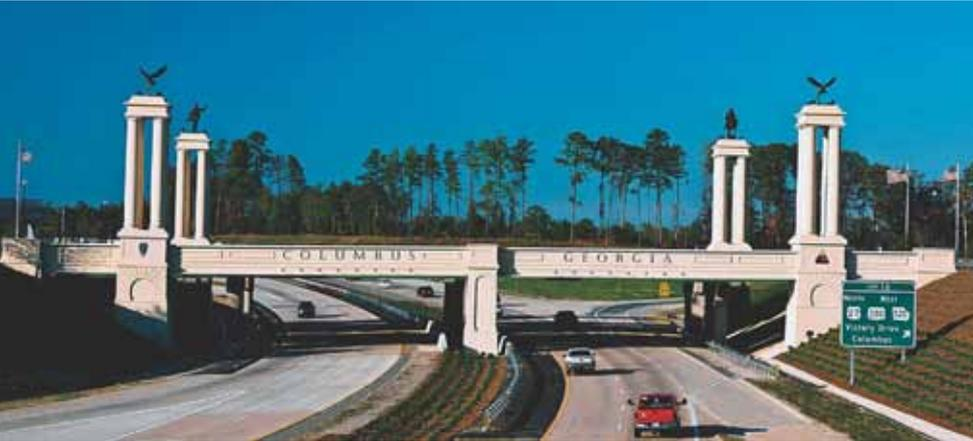
*Left: To dress up the gateway to Fort Benning, Ga., designers created freestanding precast concrete façades that hide the existing steel bridge and added a precast concrete column pedestal at each corner topped with a bronze statue.*
