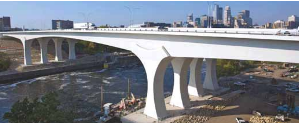
The new I-35W Bridge across the Mississippi River in Minnesota provides continuity throughout the bridge and state-of-the-art smart bridge technology that monitors bridge behavior in real time. Photo: FIGG Bridge Engineers.
