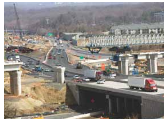
I-495 Capital Beltway Express Lanes construction.
