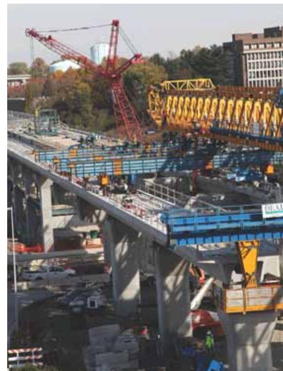
Metrorail construction at Tysons Corner, Va.
