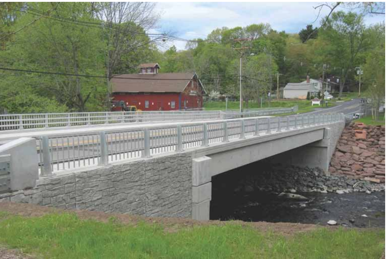
The South Maple Street Bridge in Enfield, Conn. Photo: Hoyle, Tanner & Associates Inc.
