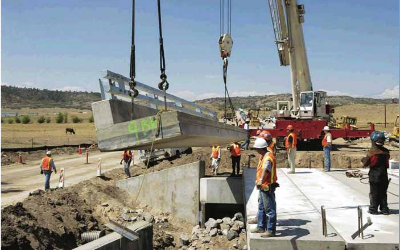
The State Highway 86 Bridge over Mitchell Gulch in Colorado.
