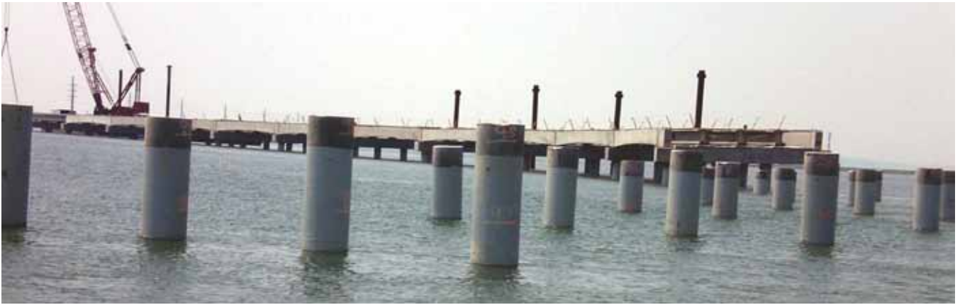
The substructure consisted of 36-in.-diameter cylinder piles. Photo: Hardesty & Hanover.
