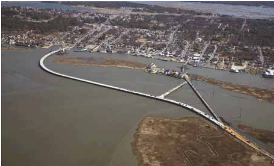
Aerial view of the new Chincoteague Island Bridge site. Photo: Patrick J. Hendrickson.
