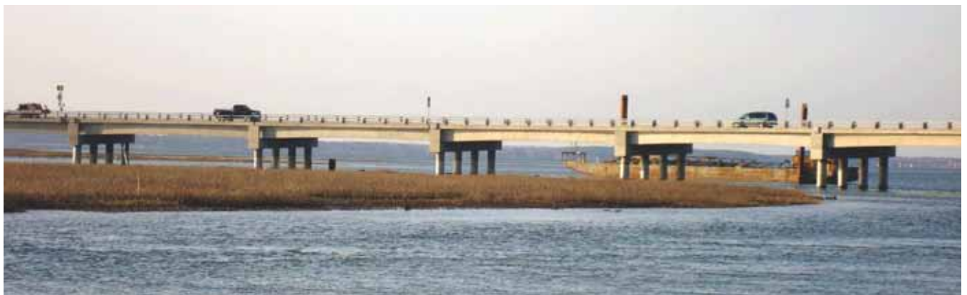
The new Chincoteague Island Bridge elevation. Photo: Virginia Department of Transportation.
