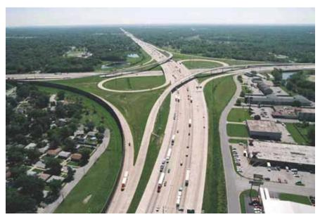
The new directional interchange on I-80/94 at SR 912 in Indiana includes 18 bridges, 8 new ramps, and all new signs and lighting.
