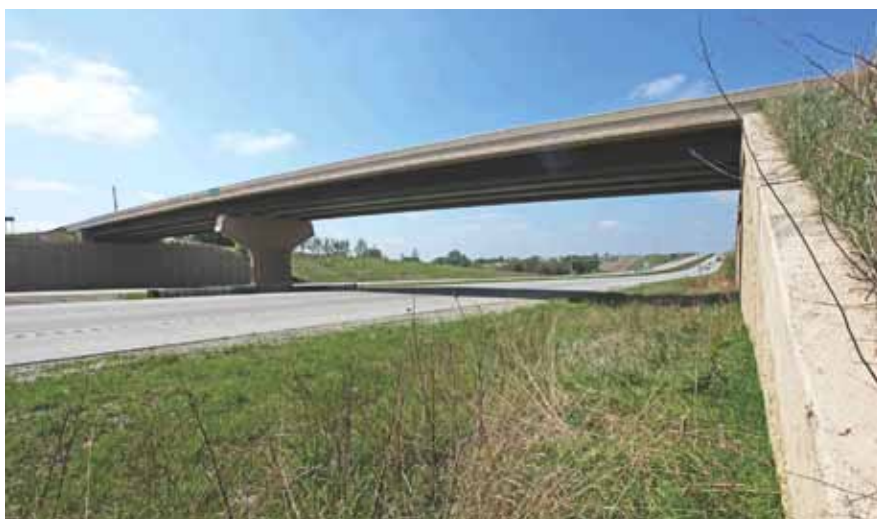
A typical NU girder bridge overpass over I-80.
