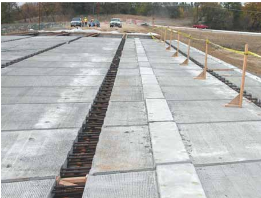
NUDECK being installed over the Skyline Bridge near Omaha, Neb.
