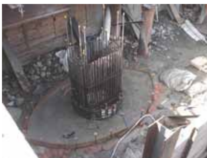
Drilled shaft to arch rib connection bars at bent 3.
