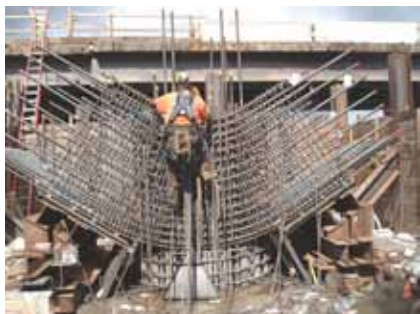
Placing rib cross-ties through bent 3 joint.
