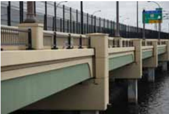
The Authority has used Florida U-beams as an economical alternative to steel box girders. Photo: Orlando Orange County Expressway Authority.
